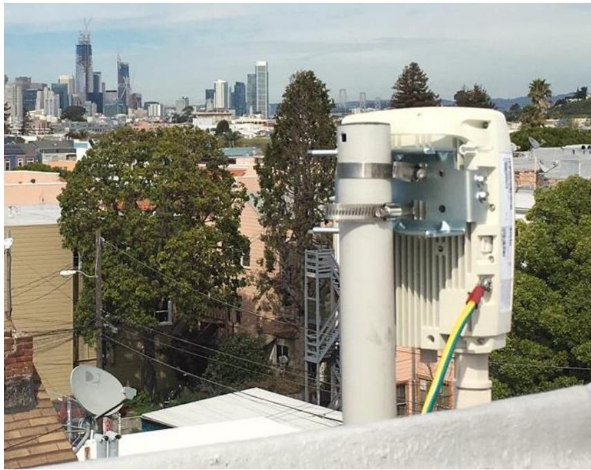
Figure 3: MultiHaul™ B100 installed
